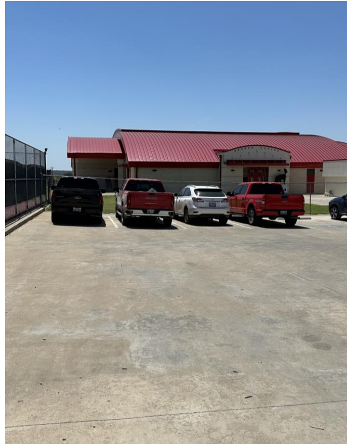
Needs pavement marking for fire lane
